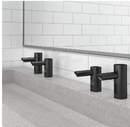
Touch-free Faucets Soap Dispensers Toilets and Urinals
