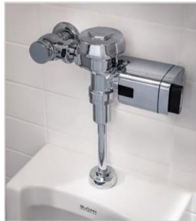
Side-mount Operators (SMO's) – battery-powered bolt-on kits to upgrade manual toilets and urinals to sensor operation
